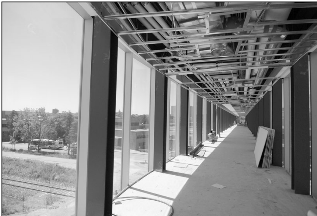
Inside the Engineering 5 link looking towards the Engineering 3 Tower
