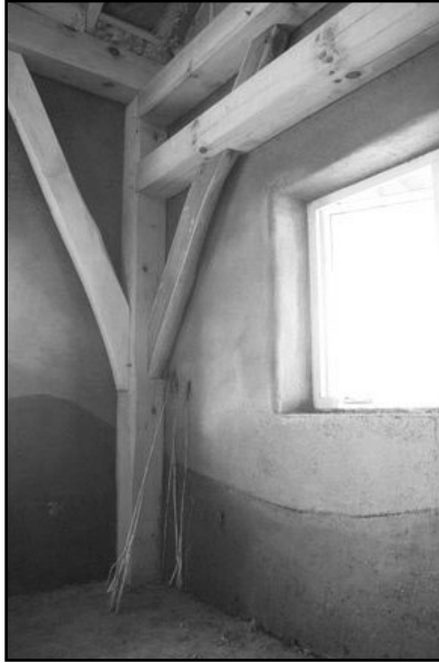
A finished first coat of earthen plaster.
