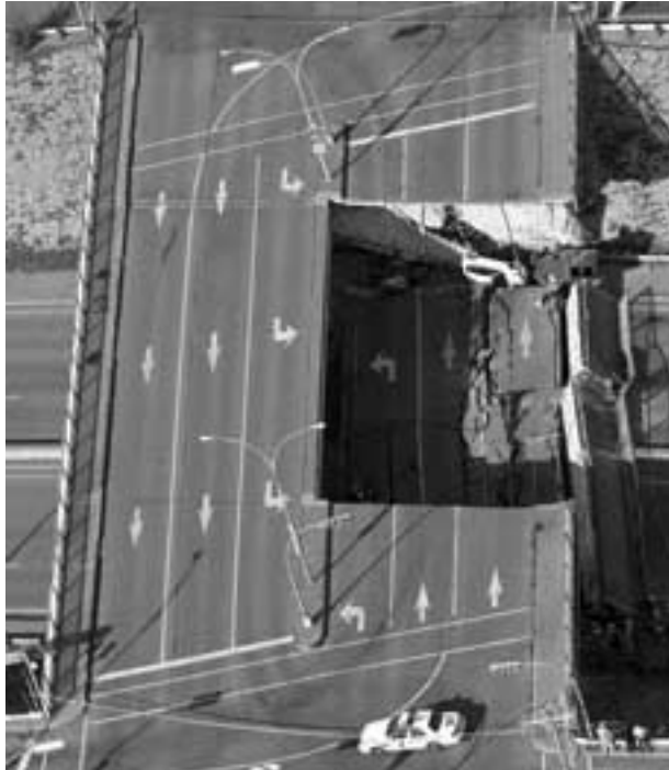
Top View of the Collapsed Overpass
