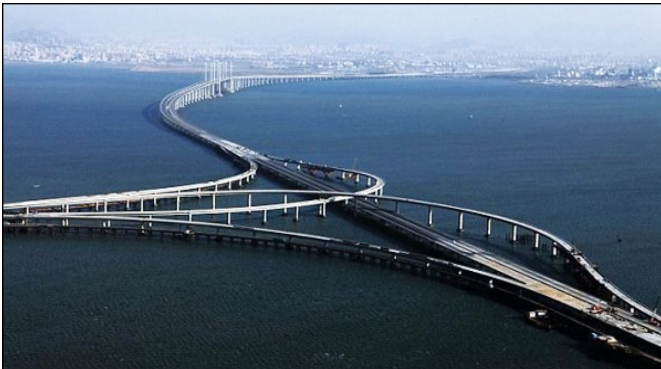
Qingdao Haiwan Bridge, which took four years to build and opening in 2011.
