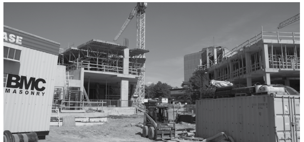
Buildings going up fast at the Science Teaching Complex
