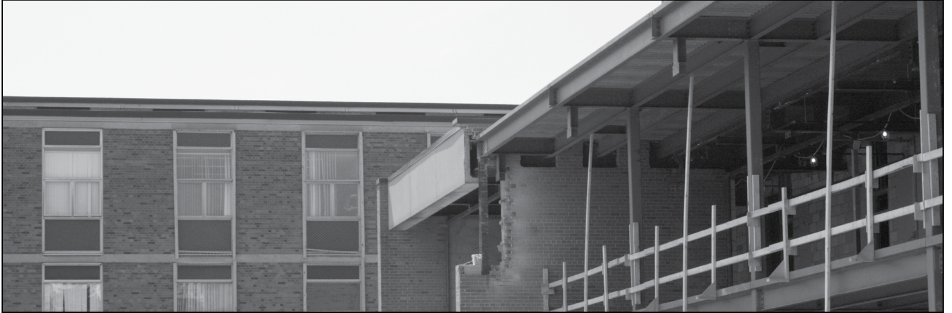
Waterloo's oldest engineering building is undergoing major renovations in the C-Wing.
