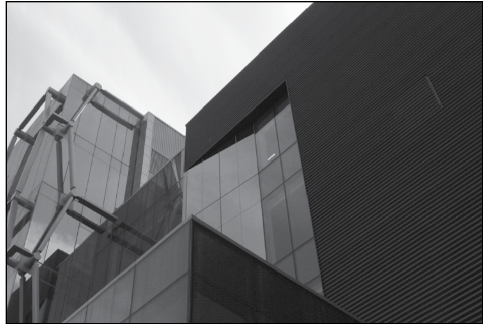
The Quantum Nano Centre is nearing completion.
