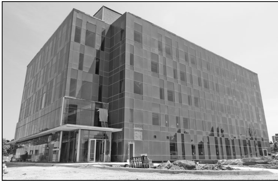
Engineering 6 Under Construction
