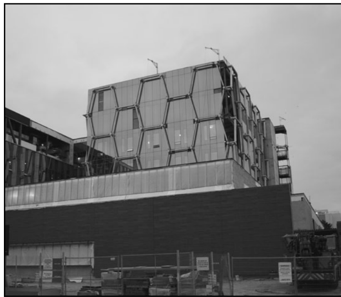
Quantum Nano Centre Under Construction
