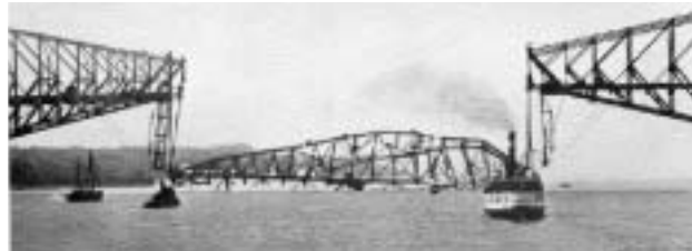
The Québec Bridge after its center span collapsed in 1916, killing 11 more workers.
