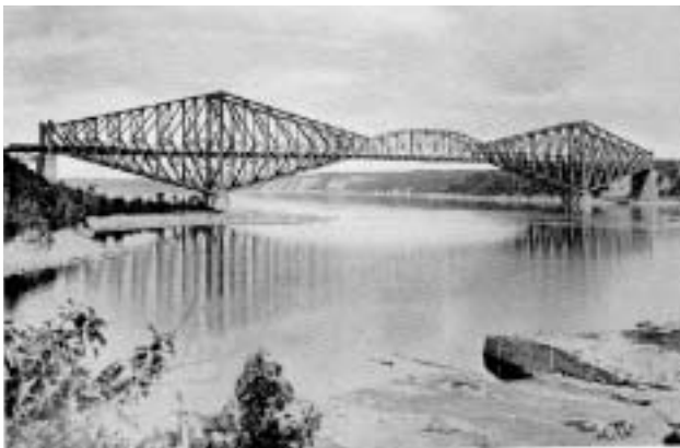
The completed Québec bridge as it stands today.
