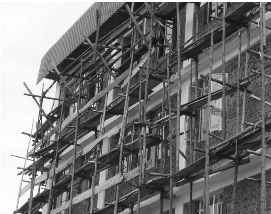
Scaffolding on a 5-story building in Kampala, Uganda.
