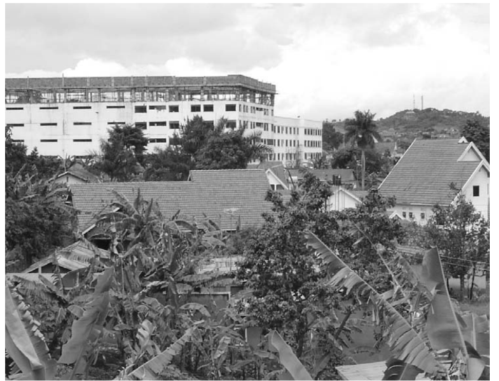
Construction on a Ugandan building
