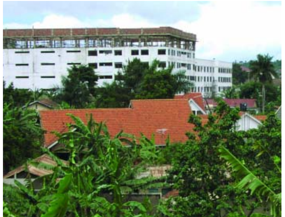
Halted construction on Kampala International University
